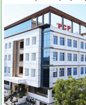
PCP Sikar : Piprali Road (Campus - 1)
