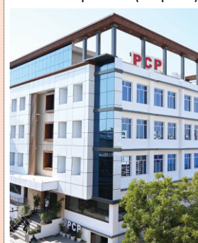
PCP Sikar : Piprali Road (Campus - 1)
